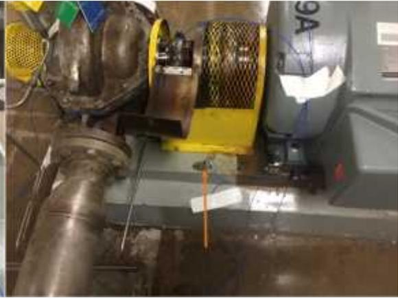
Figure 7: Base Between Bolts Accelerometers
