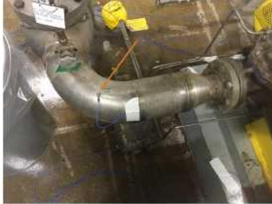
Figure 10: Discharge Elbow Accelerometer
