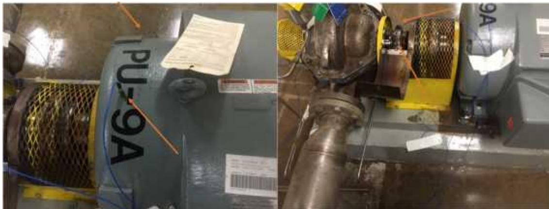
Figure 4: Inboard Motor Accelerometers      Figure 5: Inboard Pump Accelerometers
