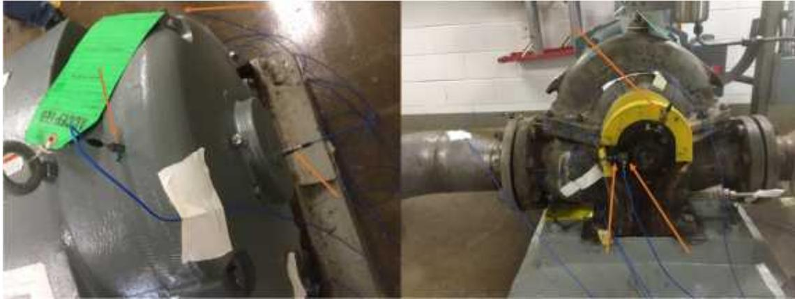
Figure 2: Outboard Motor Accelerometers      Figure 3: Outboard Pump Accelerometers
