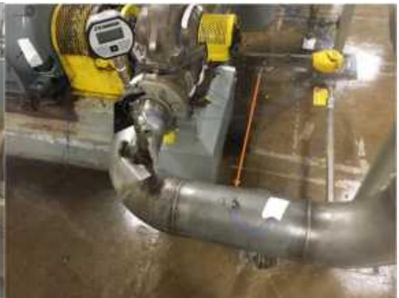
Figure 9: Suction Mid-Pipe Accelerometer
