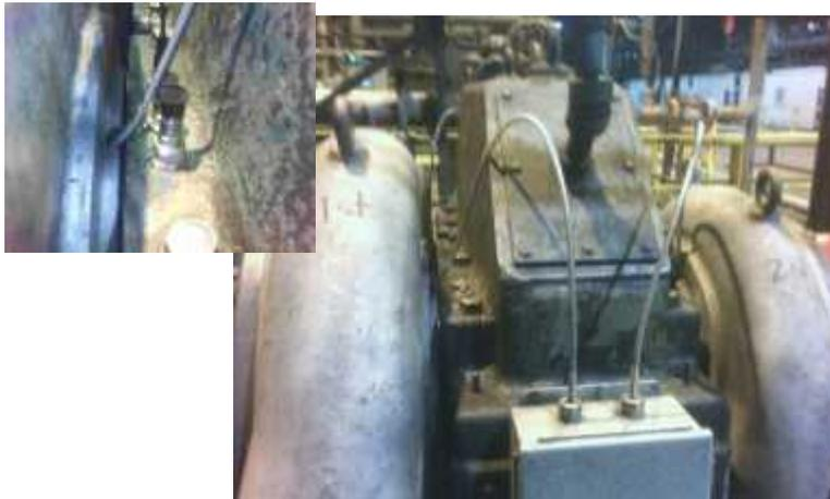
Figure 9. Centrifugal compressor
